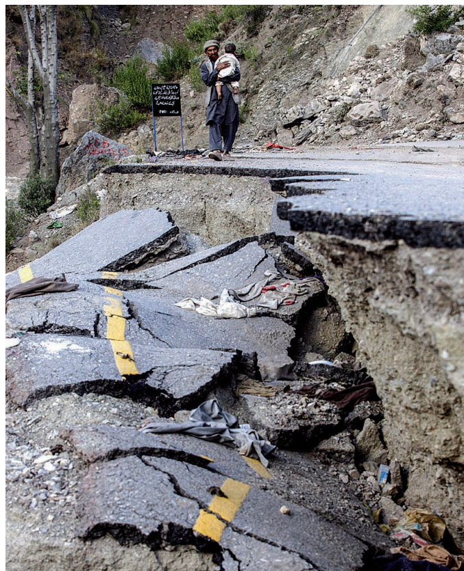
Damage done by a 2005 earthquake in Balakot, Pakistan
